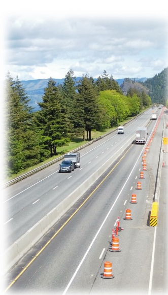
Concrete barriers moved to I-84 East bound lanes
