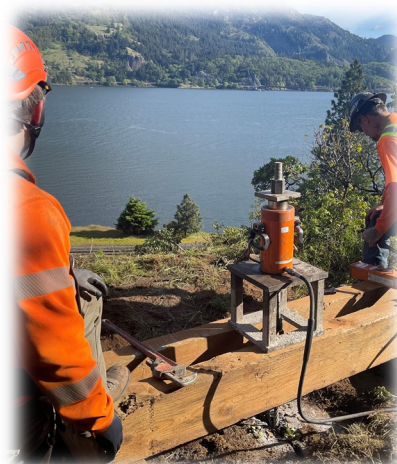
Wire mesh anchors testing
