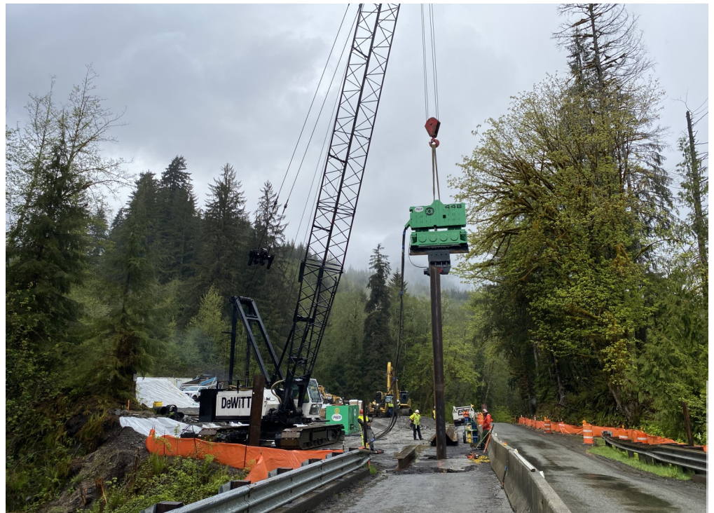
ICl subcontractor installing temporary sheet pile shoring
