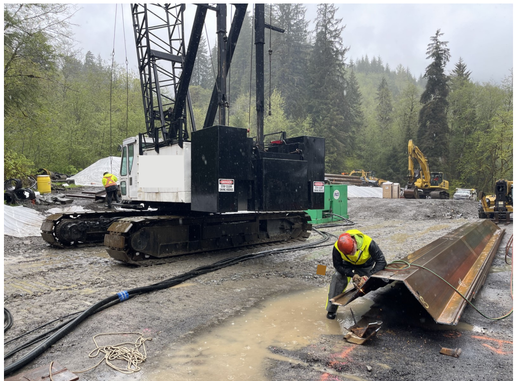
ICl subcontractor preparing equipment for temporary sheet pile shoring
