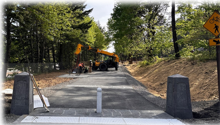
Installation of pilasters & signs
