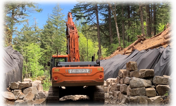
Big Cut rockery wall
