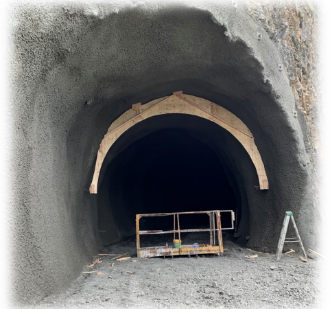
Form work East tunnel portal
