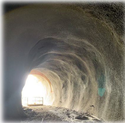
Left: Finished steel fiber reinforced shotcrete at East Portal
