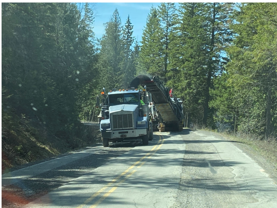
Milling existing asphalt on the Going to the Sun Road.
