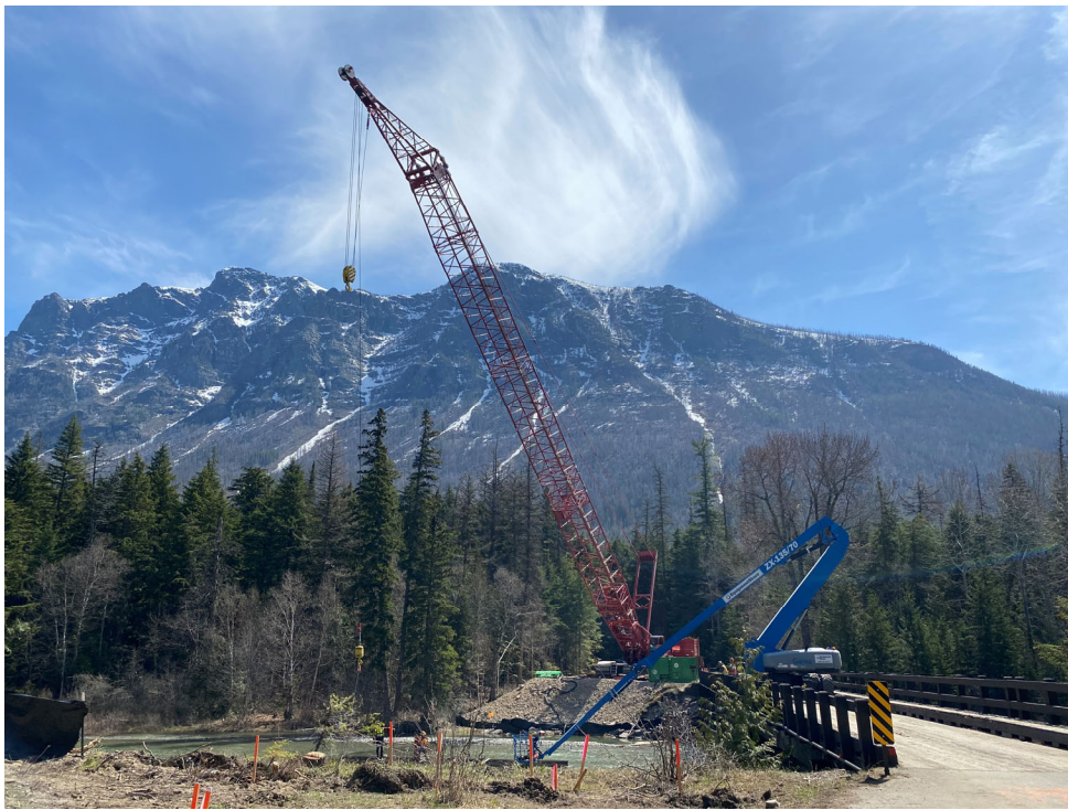
440 ton Crane setup on pad setting up for pile driving operations.
