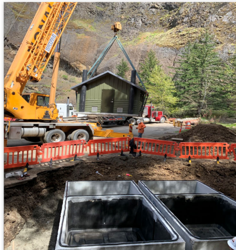
Below: Pre-Fabricated Vault Toilet Installation
