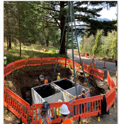
Below: Pre-Fabricated Vault Toilet Installation
