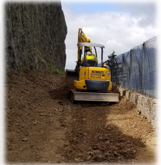
Clearing and grubbing operations
