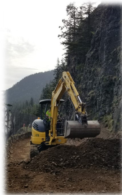
Clearing and grubbing operations
