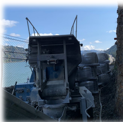
Below: Shotcrete batch equipment set up
