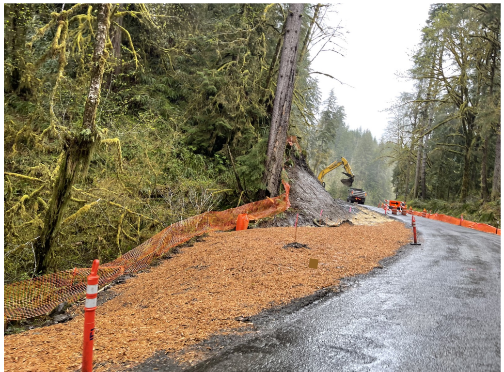
Mulch placed at Tower Creek for erosion protection
