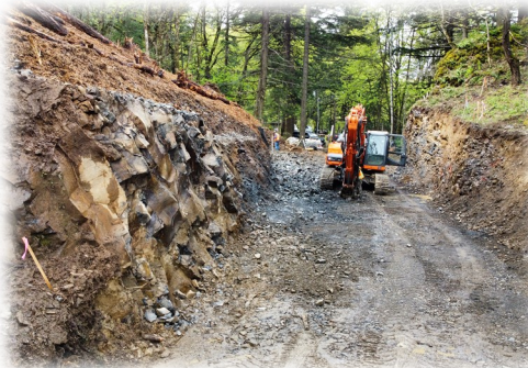
Contractor finishing excavation at Big Cut Wall
