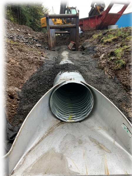
Below left and right: Culvert installation
