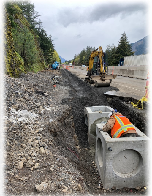
Below left and right: Culvert installation
