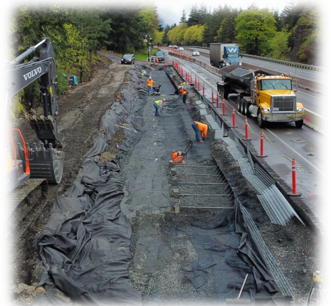
Contractor building Mechanically Stabilized Earth Wall at Dome
