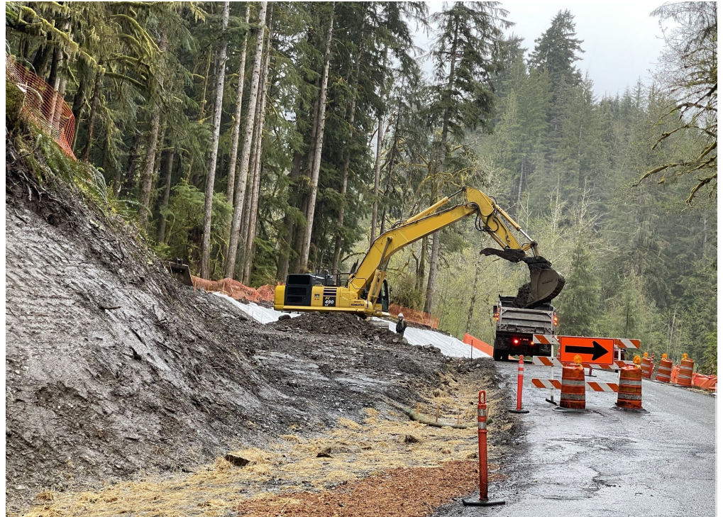
ICI excavating embankment for realignment of new road at Tower Creek
