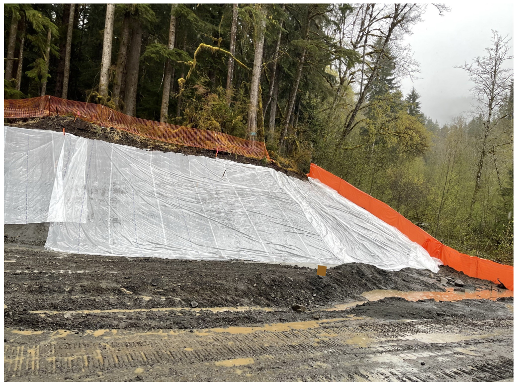
ICI covering slopes to protect against erosion
