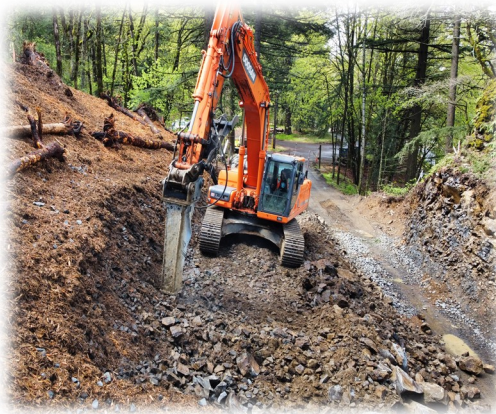
Contractor excavating at Big Cut Wall
