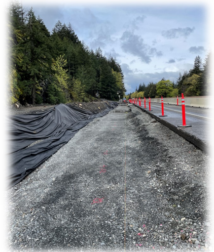
Contractor preparing foundation for Mechanically Stabilized Earth Wall at Dome Rock
