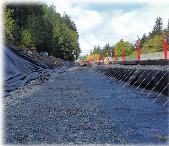
Below: Mechanically Stabilized Earth Wall at Dome Rock
