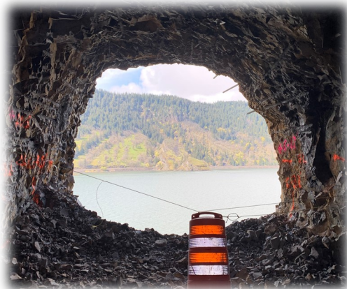
Below and Right: Adit #3 & #4 mechanical excavation
