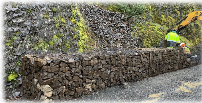
Construction of Gabion baskets
