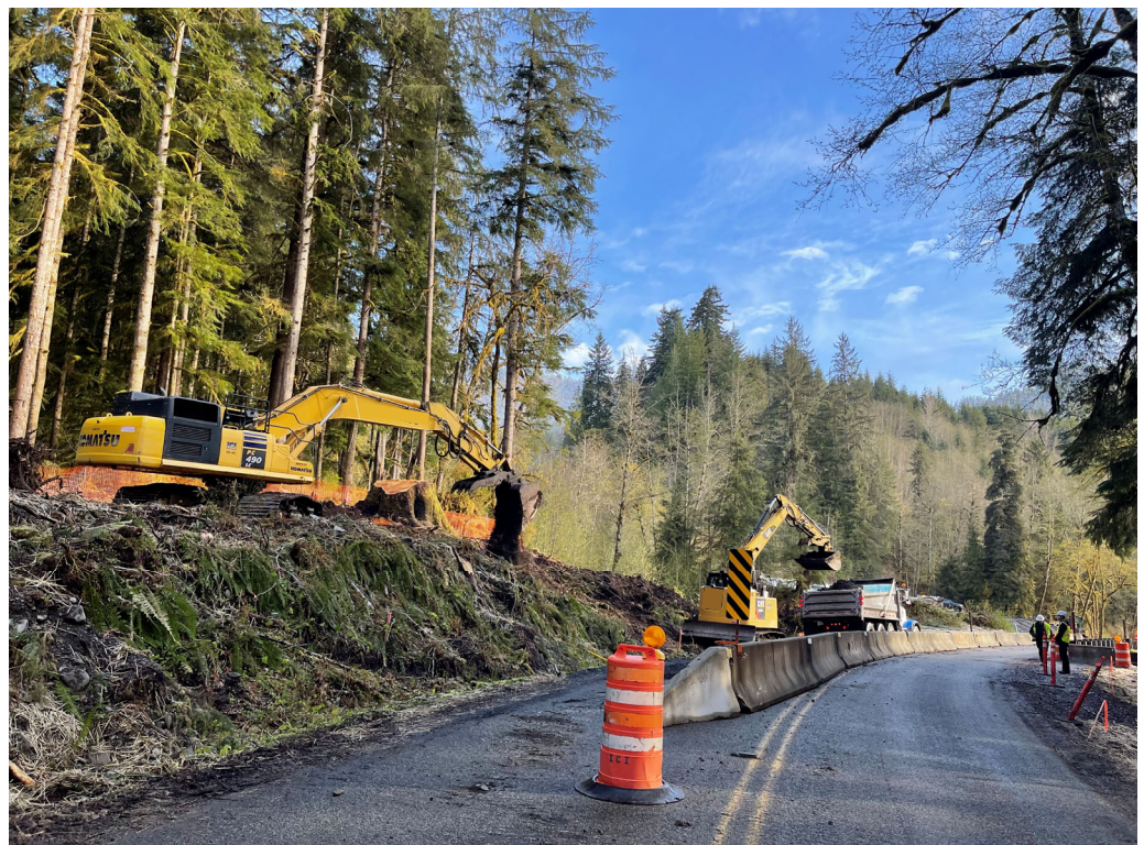
ICI excavating embankment for realignment of new road at Tower Creek
