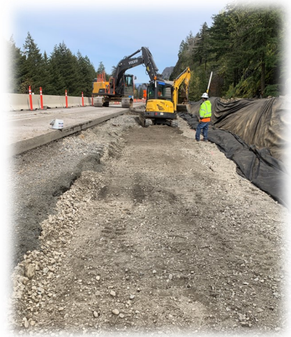
Contractor preparing for Mechanically Stabilized Earth wall
