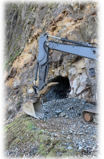
Right: Adit #1 exterior
