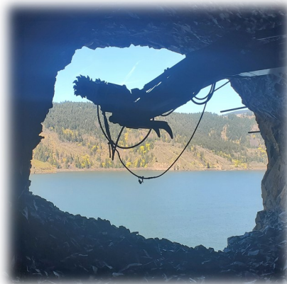
Below: Adit #3 portal view
