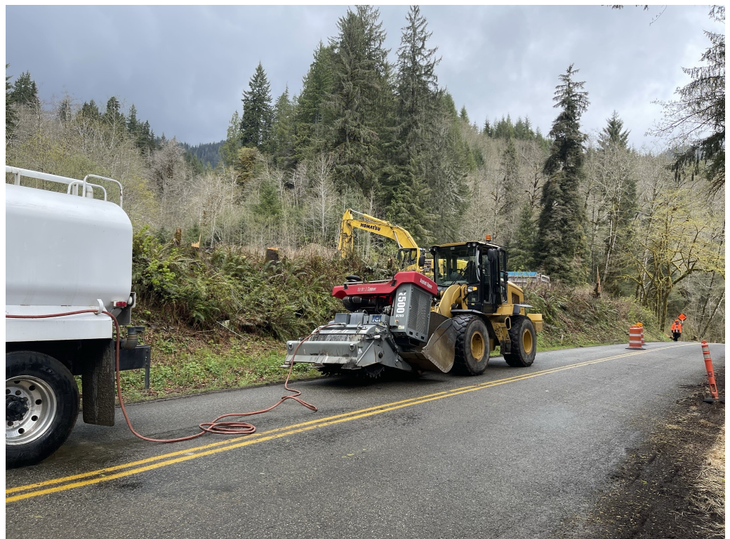
Milling north lane on east approach to Tower Creek
