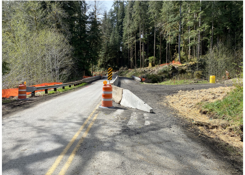
Tower Creek bridge traffic shifted to south lane
