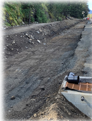
Installation of storm drain
