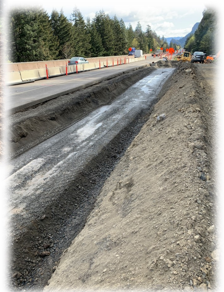
Preparing the foundation for Mechanically Stabilized Earth wall
