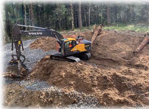
Contractor placing landscaping trees on slope
