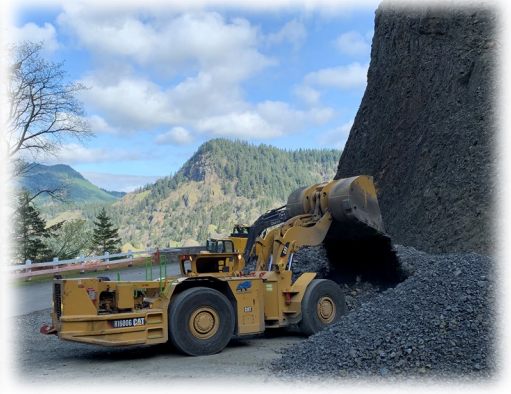
West tunnel mucking
