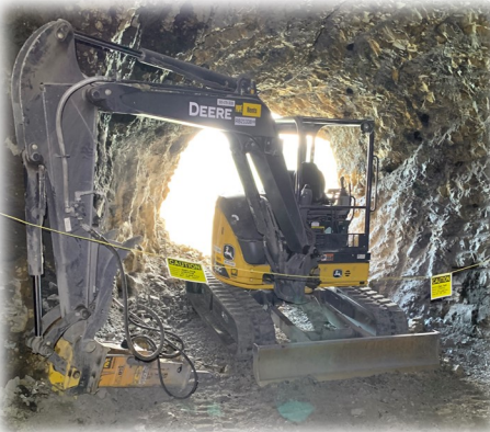
Adit 4 mechanical excavation
