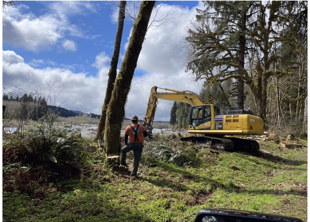
Clearing trees at MP 3-4 at wetland mitigation site
