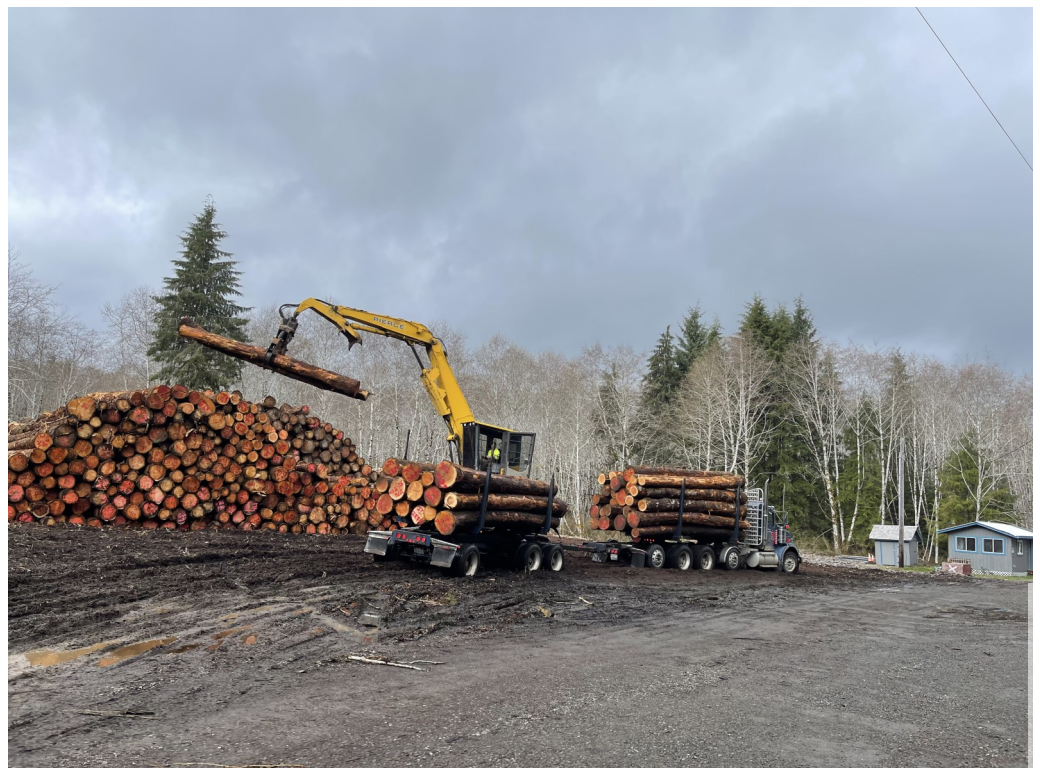
Stockpiling logs for use in the Engineered Log Jams
