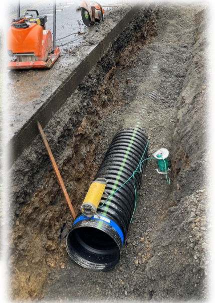
Storm drain installation
