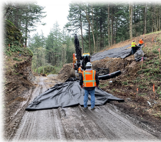
Geotextile material placement on the backslope of the Big Cut wall
