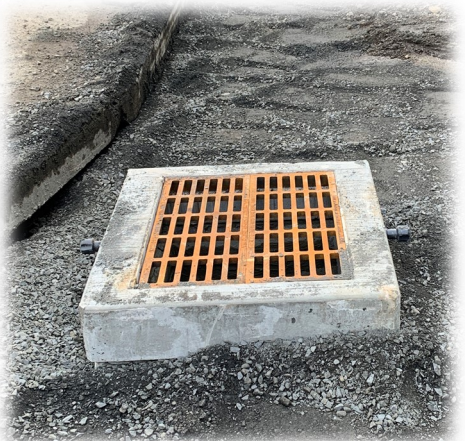
Storm drain installation
