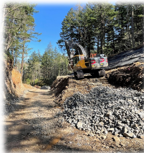
Drain rock being placed on the Big Cut wall
