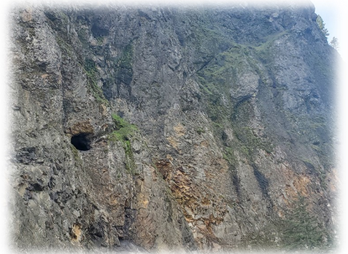
Adit 4 exterior view
