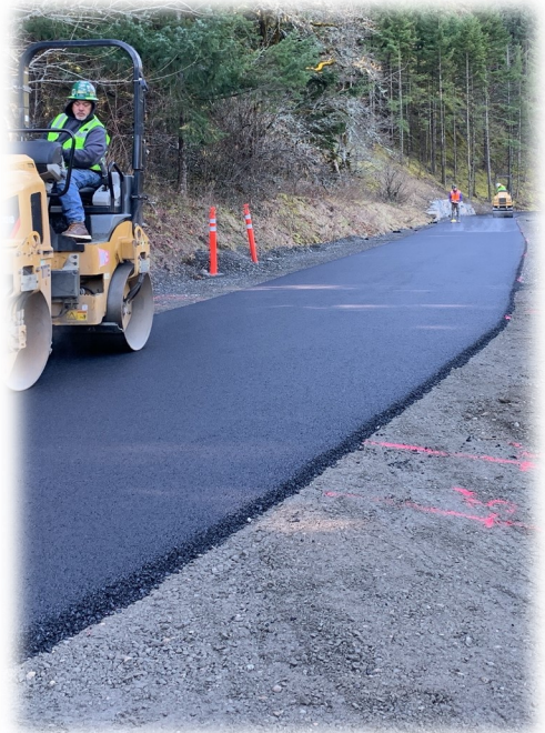
Compacting asphalt pavement
