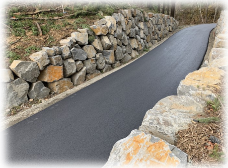
Above: New asphalt
