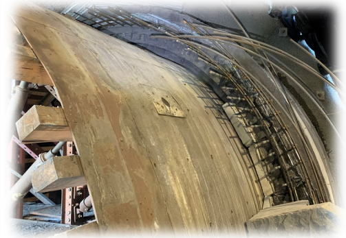
Below Left & Right: East tunnel portal arch structure concrete forming
