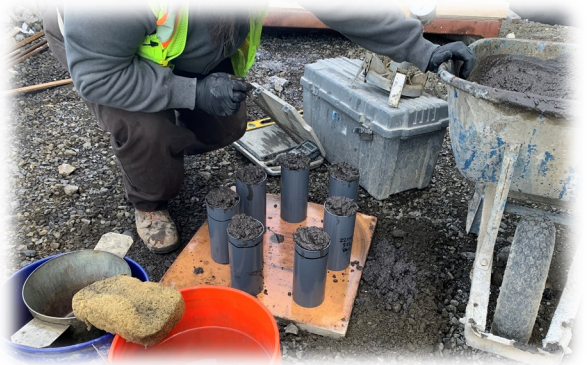
Below: Concrete sampling
