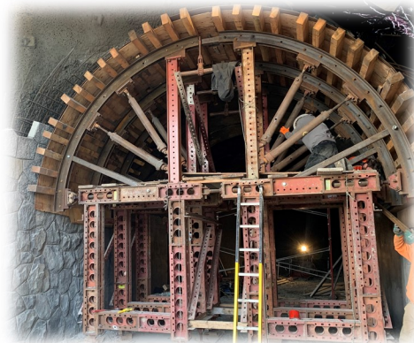
Below Left & Right: East tunnel portal arch structure concrete forming
