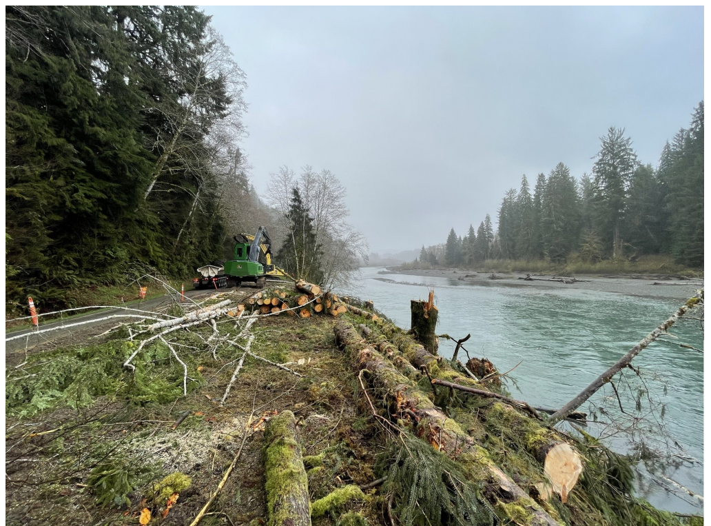
Clearing trees at MP 4 along river bank where ELJs will be installed
