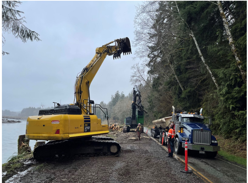
Clearing trees at MP 4 along river bank where ELJs will be installed
