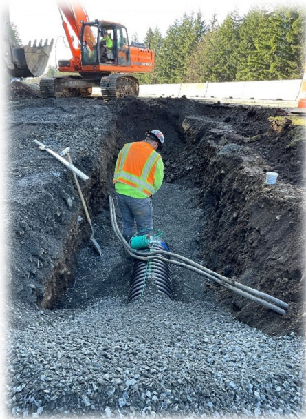
Beginning of installation of culverts
