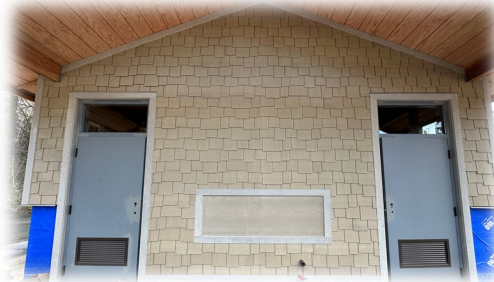
Right: Finished siding on Campground restroom
