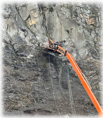
Drilling drain holes within Stepped Cut
