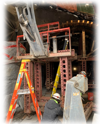
Left & Right: East portal tunnel arch concrete form support assembly
