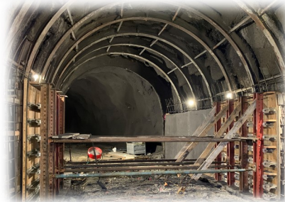
Right: West portal structure concrete wall support
