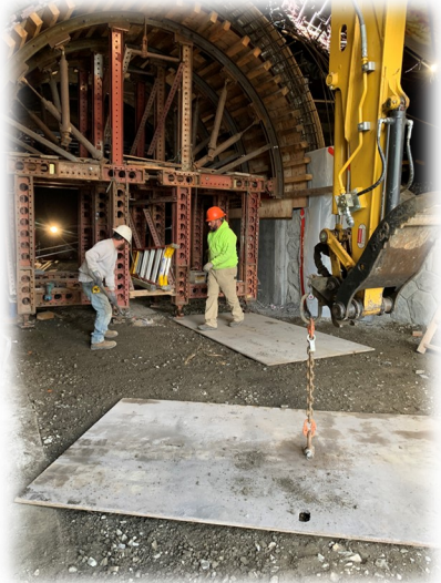
East portal structure frame form relocation
