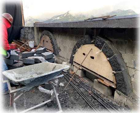
West portal wall concrete form
