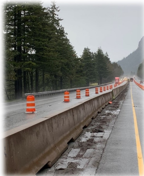
Installation of temporary median barrier rail
