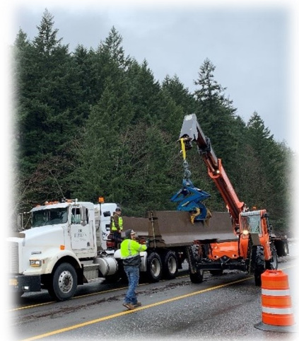
Storage of existing center median barrier rail
