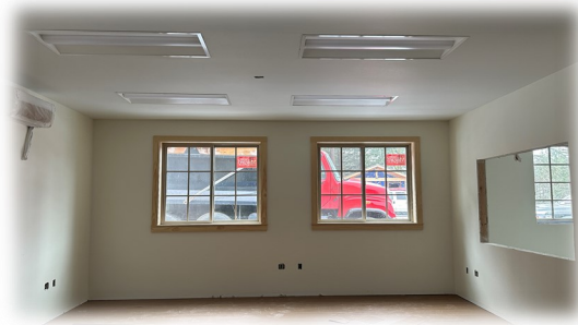
Right: Finishing work inside the Viento Maintenance Facility
