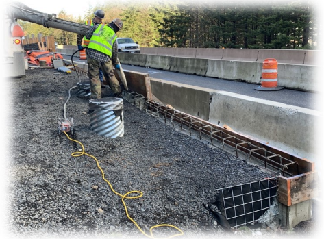
Concrete pouring at Dome Rock MSE wall
