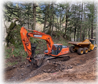
Trail excavation begins
