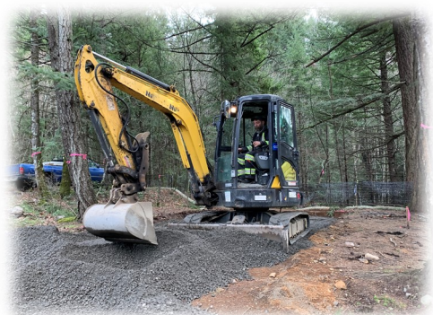
Placing aggregate base in camp site
