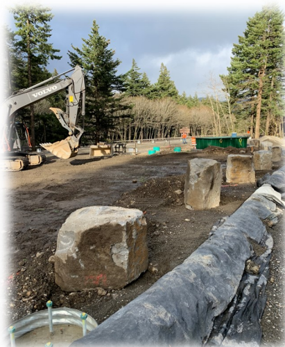
Placement of boulders at parking lot
