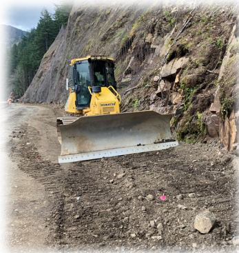
Cutting ditch at Hackly Cut
