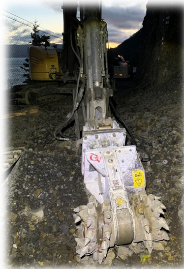
Below: Grinder attachment working at Adit #5 - Right: Barrier and attenuator intersection
