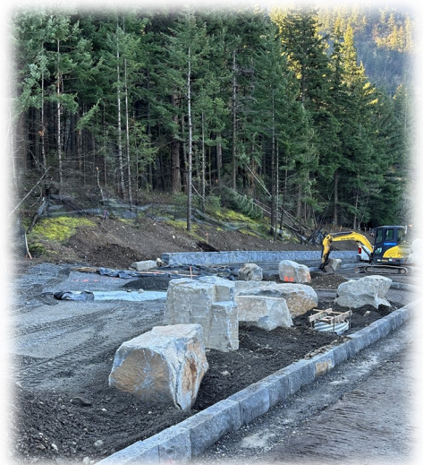
Placement of boulders at entrance
