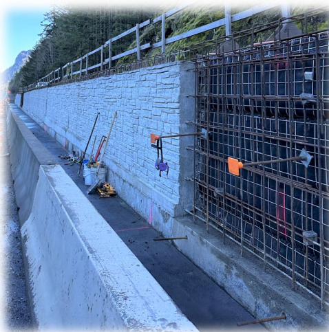
MSE wall at Ridge Cut
