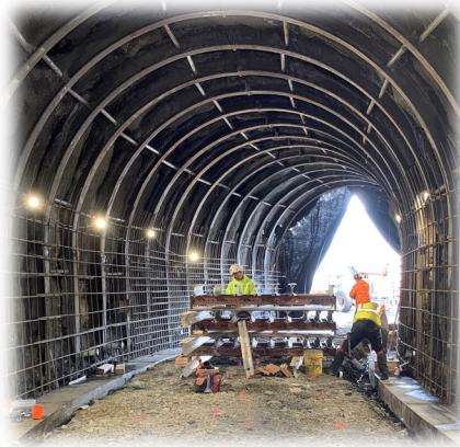
Below Left: West portal type 3 area rebar installed on South side
