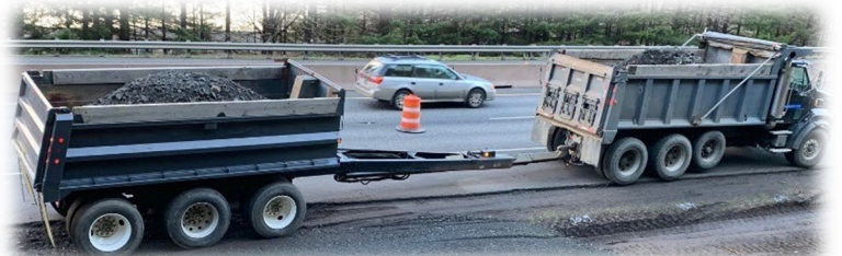
Right: Embankment material delivery
