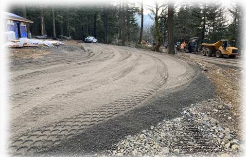
Below: Grading for Campground Loop Road
