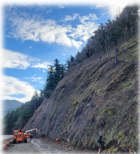
Left: Midslope Rockfall Attenuator system at Hackley Cut
