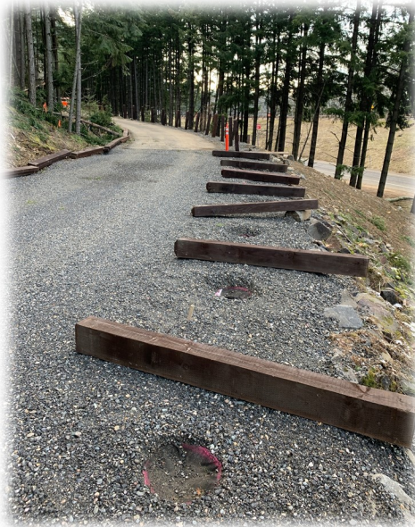
Fence posts for Pedestrian Railing
