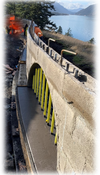
Left and Right: Picket infill concrete at West bench
