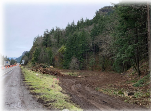
Right: Guardrail removal
