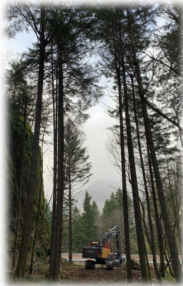
Below: Clearing and Grubbing
