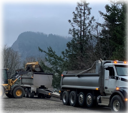
Below Left & right: Loading spoils from East staging area and stockpiling at Wyeth site.
