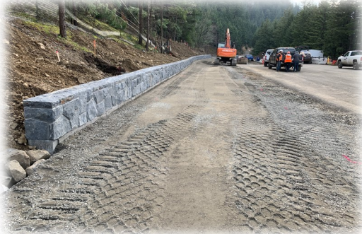
Seat wall and Trail grading
