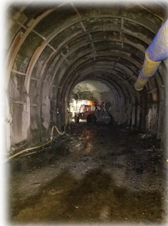
Below: West tunnel explosive loading
