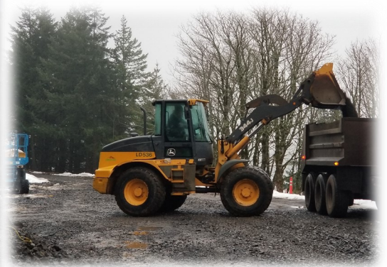
Below: West tunnel mucking to parking lot after blast loading
