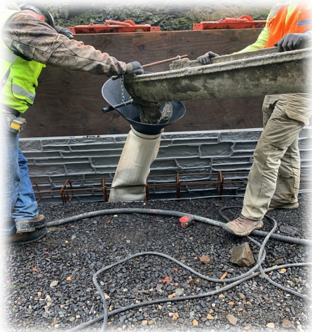
Placing concrete for Ridge Cut MSE wall
