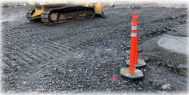
Shaping subgrade at Maintenance Facility
