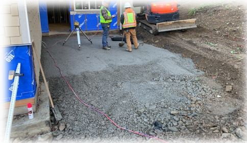
Shaping subgrade at Maintenance Facility
