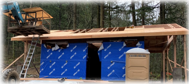
Left: Campground restroom
