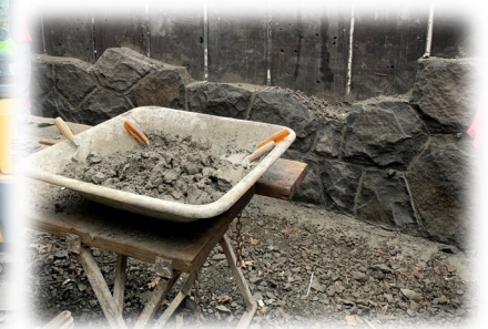
Below: East portal wing wall stone work
