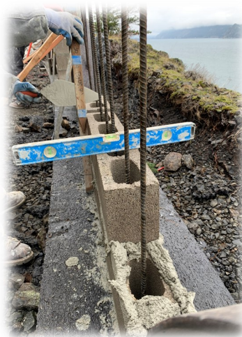
West bench Concrete Masonry Unit Wall construction
