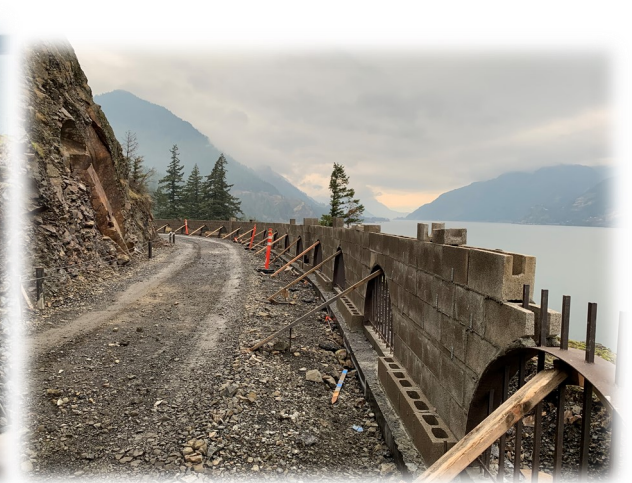
West bench Concrete Masonry Unit Wall construction
