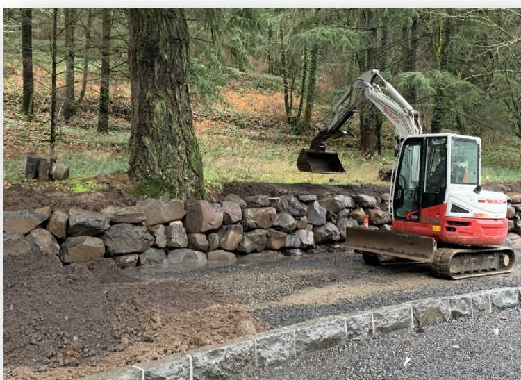
Top Soil Cover at Rockery Wall
