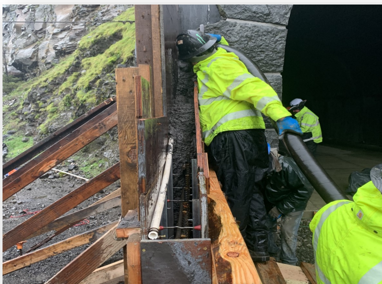
Concrete Pouring at No. Wing Wall in West Portal
