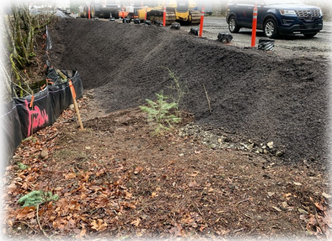
Viento Creek Reinforced Soil Slope with Placed Topsoil
