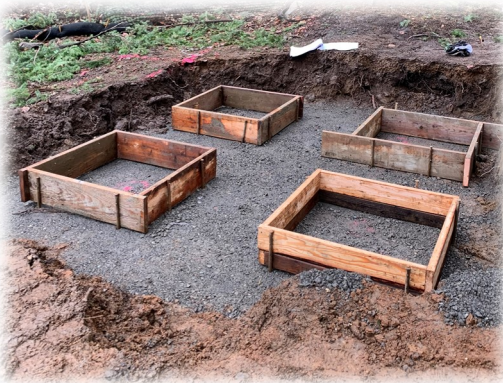
Below: Prepared Footing for Hiker-Biker Camp Pad Shelter
